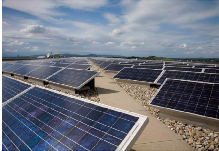
Figure 3: Grid connected PV generator on top of sic office building at Freiburg
