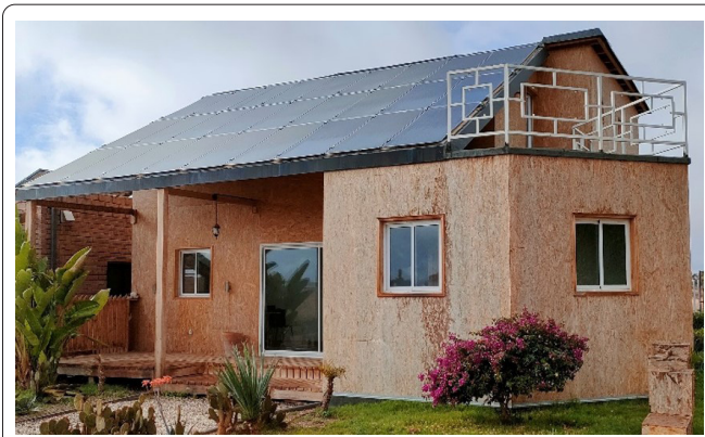
Figure 2: Case study building.
